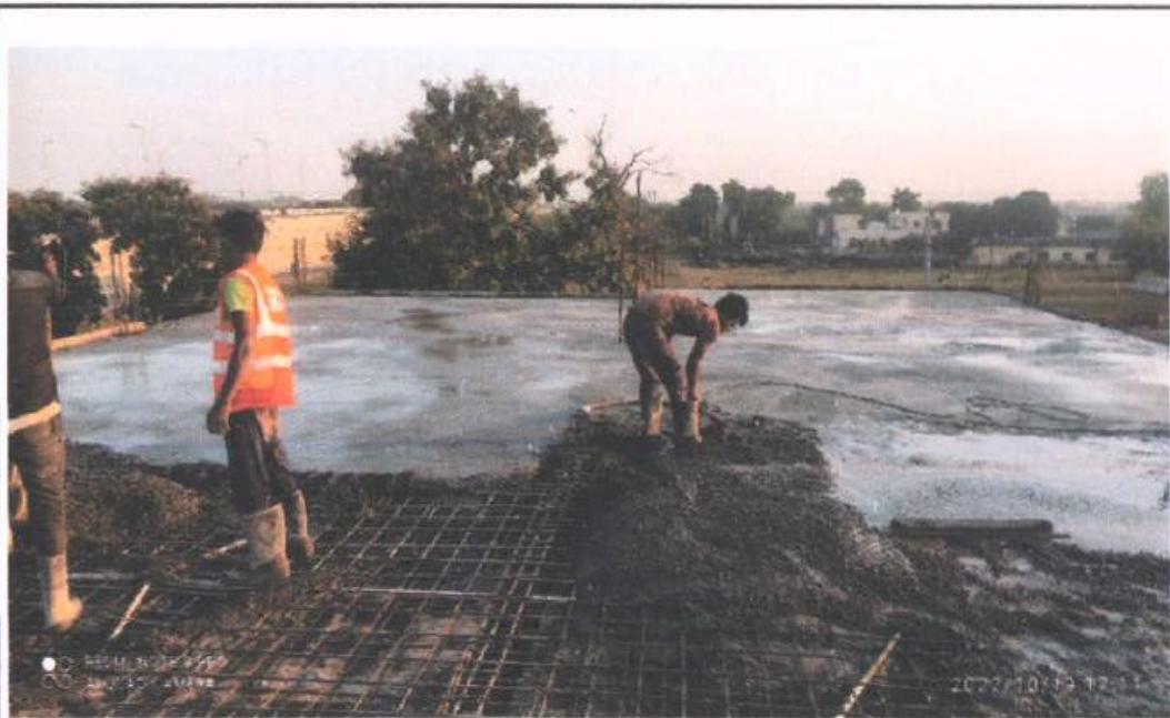
Km. 15+400 Rest Area Restaurant Block Slab Work completed RHS
